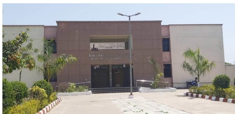
Fig 12: Secondary School in Village
