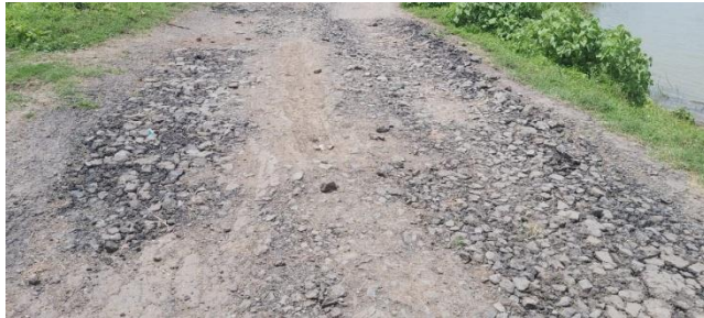
Fig 30: Road condition of Village
