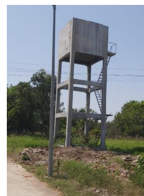
Fig 9: Overhead Tank at village
